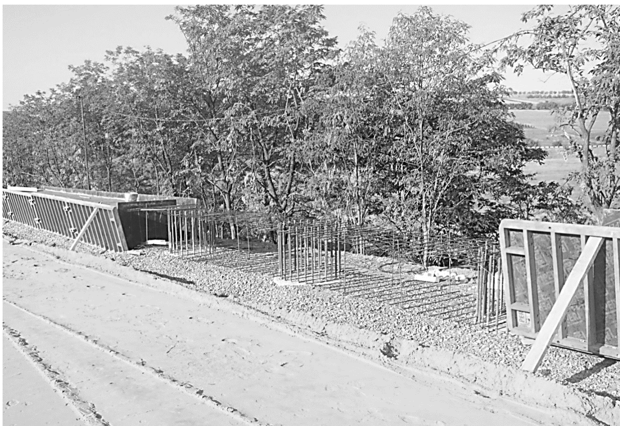
Figure 2. Arrangement of bored piles in the right slope of the embankment.
