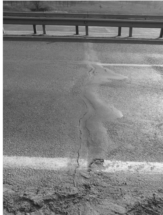
Figure 6. Transversal cracks in the road surface. December 2019.
